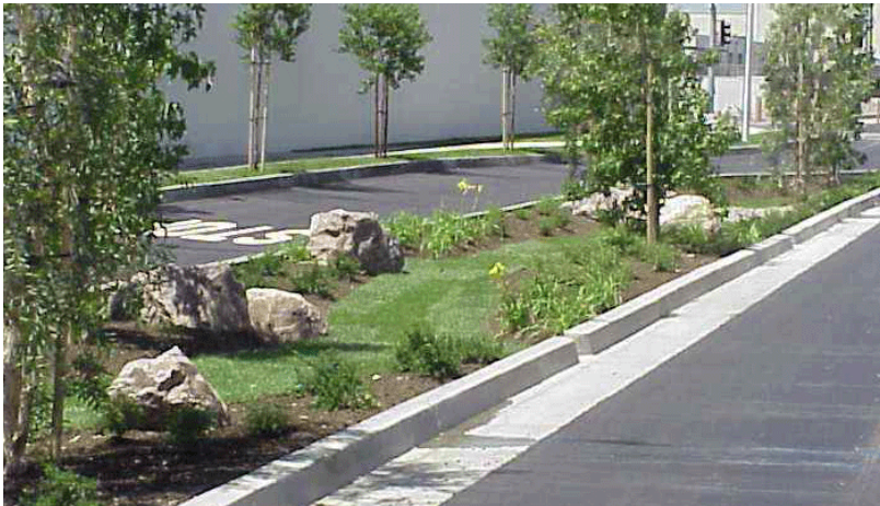
Source: Los Angeles Basin Water Augmentation Study – Neighborhood Retrofit Concept Plan Figure 33. Example Linear Bioretention Area.
